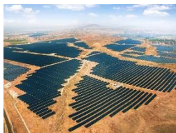
Solar Park, Rajasthan
